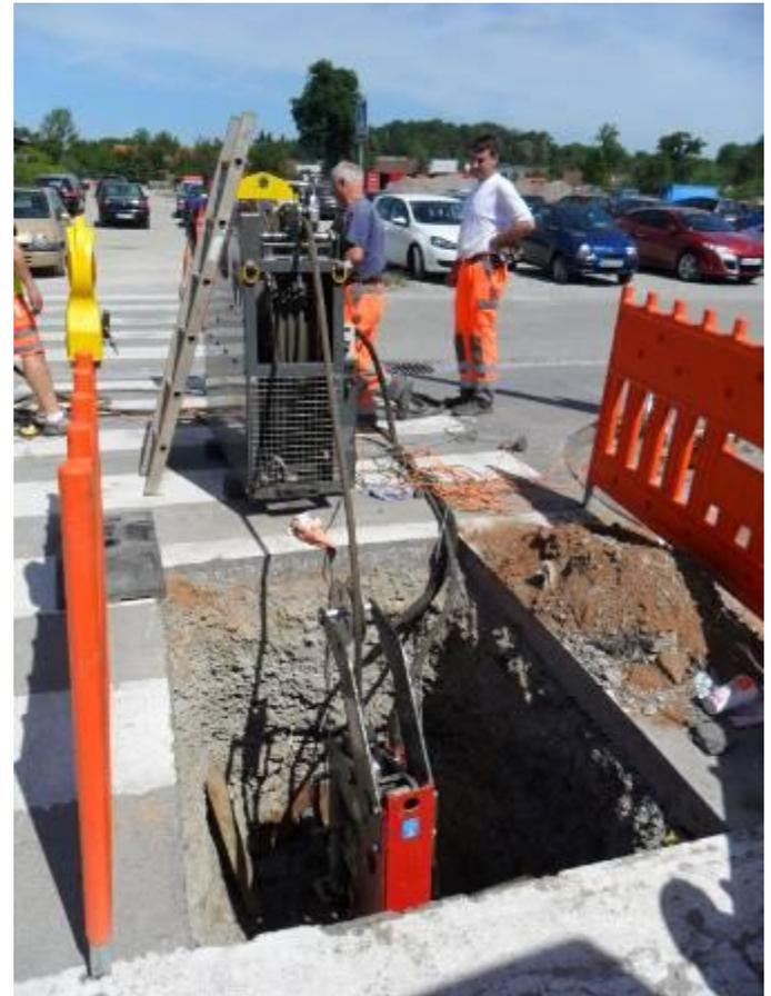
The automatic cable drum X 400 rolls the pulling cable onto the drum simultaneously with the pipe pulling.
