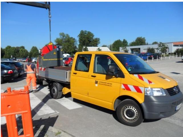
The automatic cable drum is unloaded from the truck.
