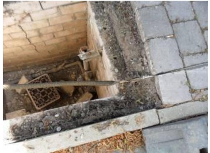
The pulling cable is pulled through the old pipe with a cable pulling sock ("Chinese finger").
