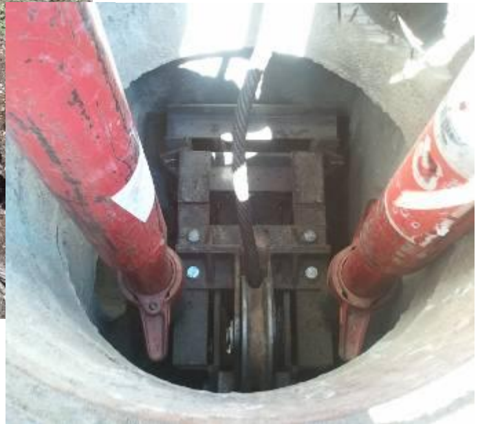
↓ The manhole frame is assembled in the manhole Ø 800 mm (32").
