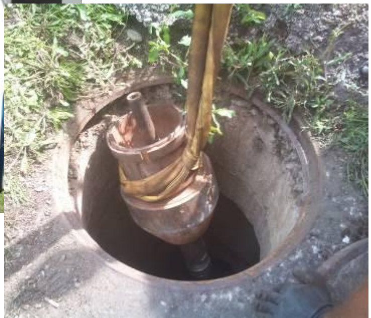
↓ The calibre head Ø 295 mm (11.6") is lifted down into the second manhole.
