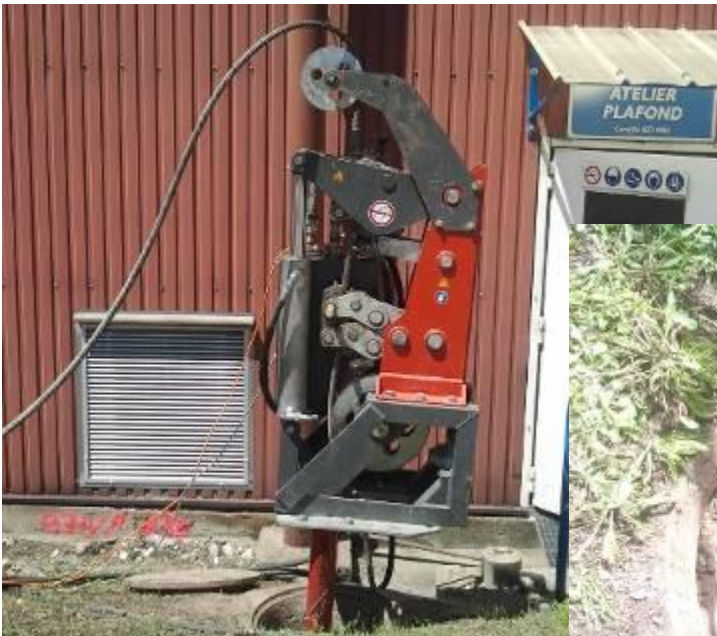
↑ The Cable Burster TERRA-EXTRACTOR X 400 is assembled via two support struts onto the manhole frame.
