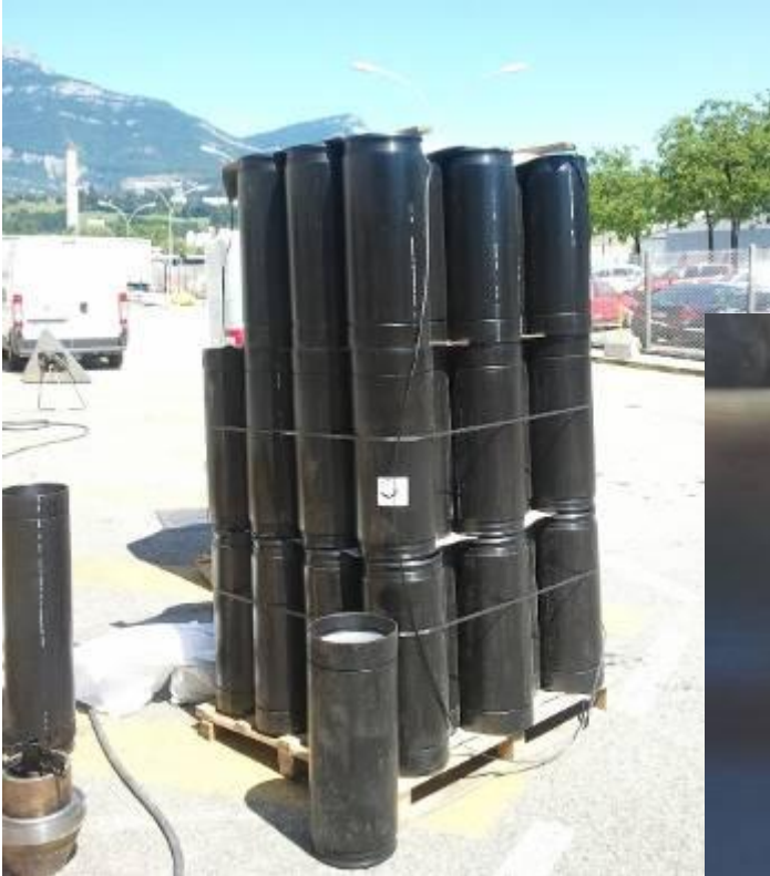
↑ These short pipes OD 280 mm (11.0") with 10.7 mm (0.42") wall thickness L = 0.70/0.64 m (27.5"/25.2") are slid into the old pipe.
