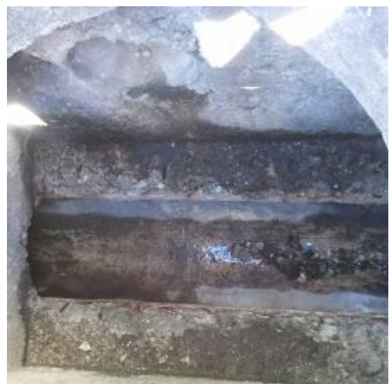
View into the manhole at the old pipe.
