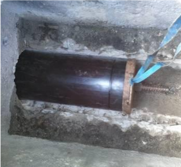
A short pipe is pulled in. This takes approximately 20 seconds.
