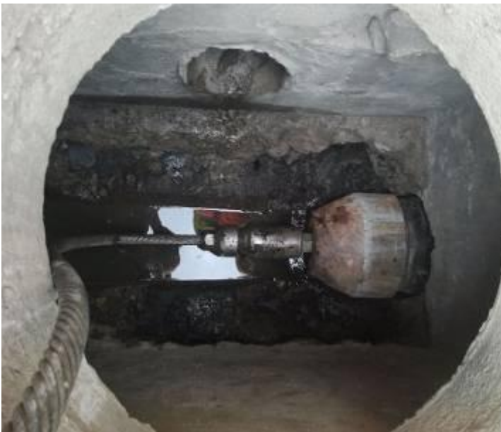
The calibre head arrives in the arrival manhole.
