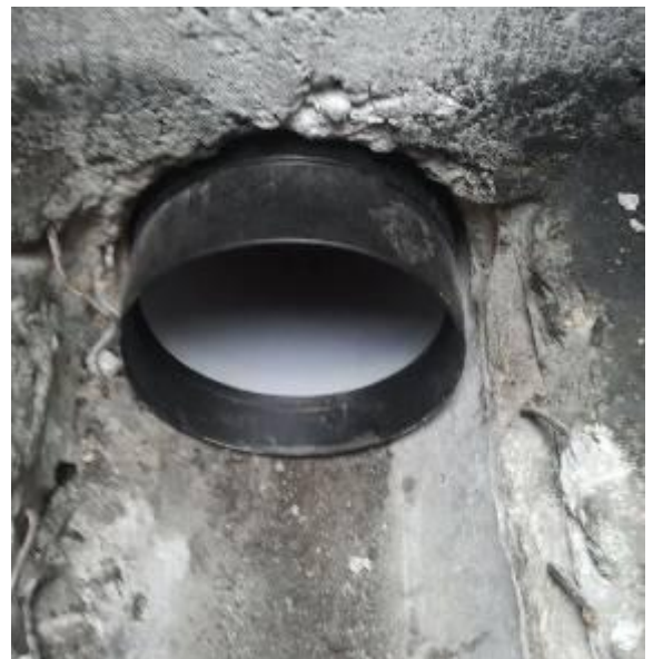
The new pipes are pulled in.
