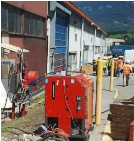
View onto one of the sections, which are to be renewed.
