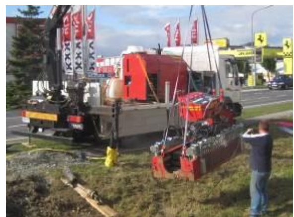
The TERRA-JET 3008 ES is cleaned after the successful bore.
