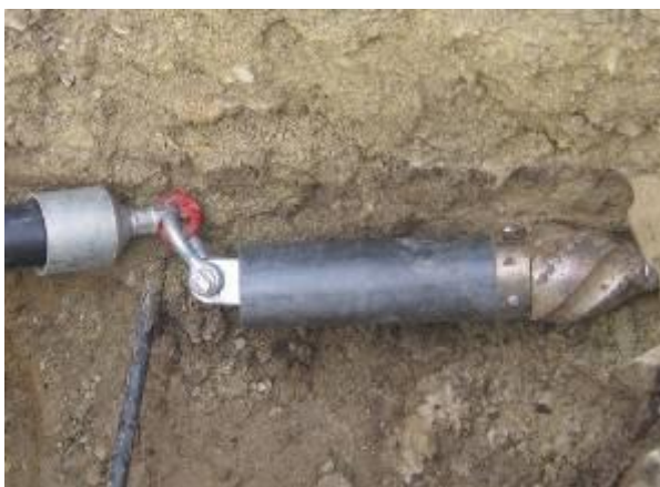
The backreamer and the new pipe just before pipe pulling.
