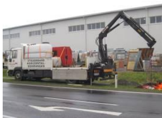
The TJ 3008 ES is lifted into the pit.
