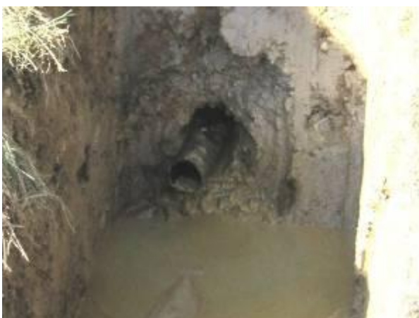
The pipe has been pulled in.
