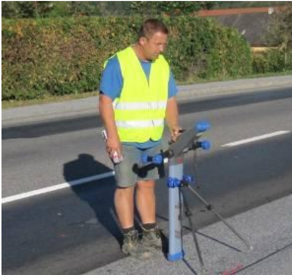
The drill head is located during the pilot bore.
