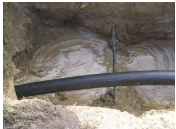
Bentonite mud comes continuously out of the bore hole during pipe pulling.
